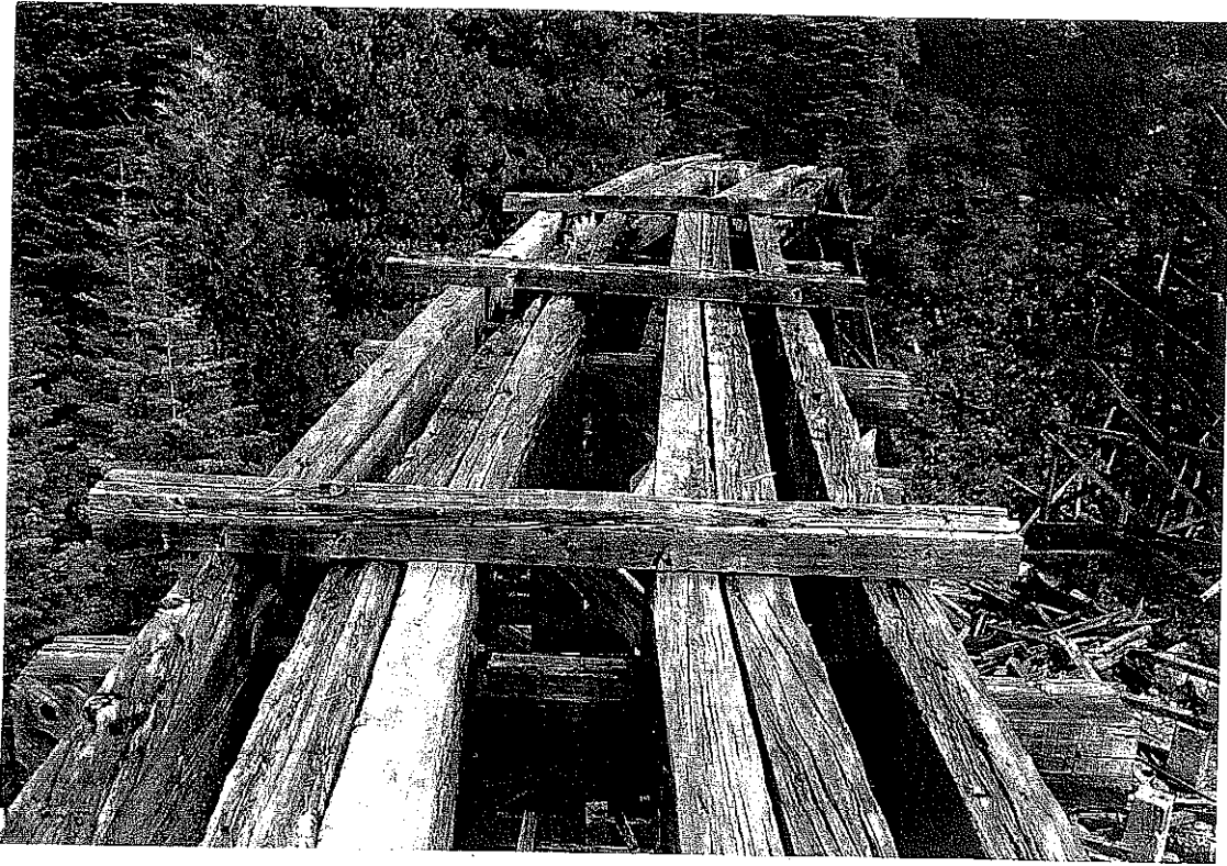
Dry rot shown on tops of stringers, heavy damage shown on stringer #1
